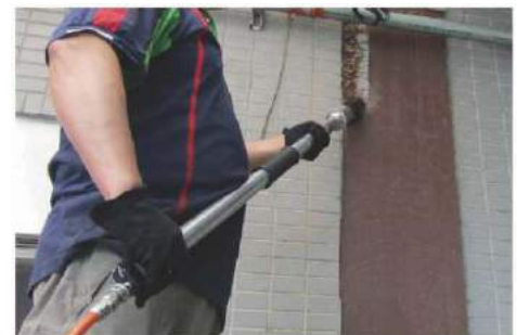
Corrosion removal for inaccessible area
